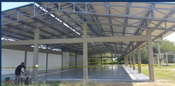
FACHADA PRINCIPAL ZONA LOBBY
